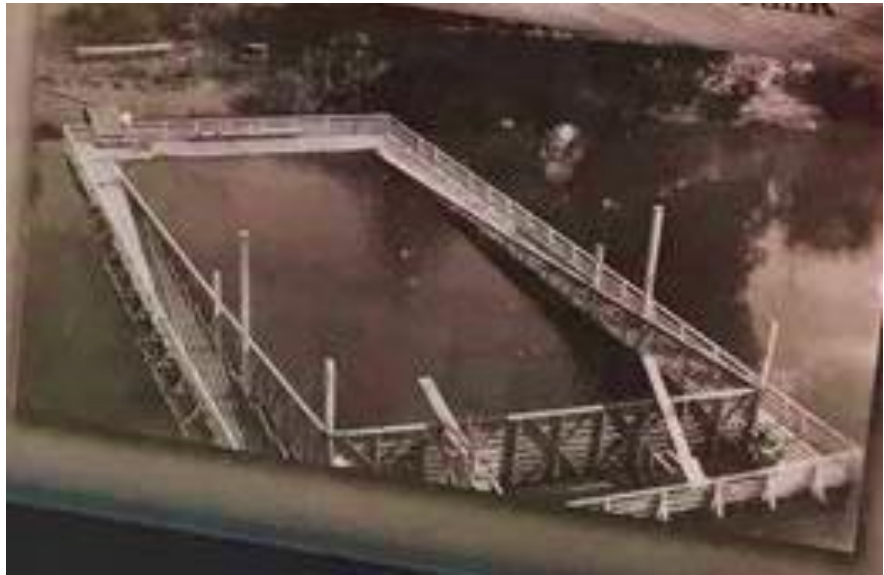
The swimming tank under construction
